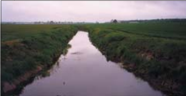
Many Eastern Shore streams, like Beaver Dam Ditch in Queen Anne's County, were channelized and deforested for agricultural drainage, which can negatively affect the stability and ecology of the system.
