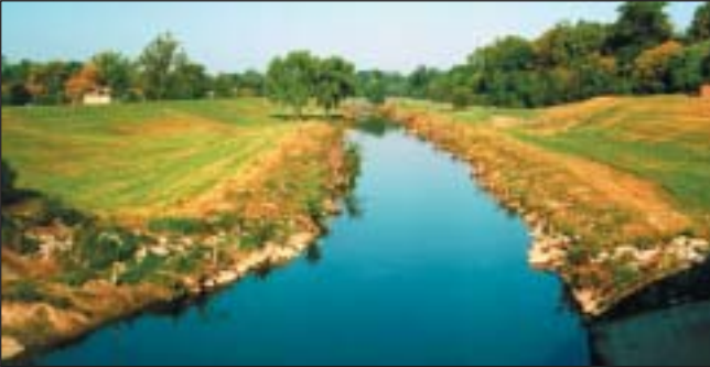
Northeast Branch in Prince George's County has been channelized with levees in order to promote the rapid movement of flood flows downstream within a narrow corridor with little hydraulic resistance.
