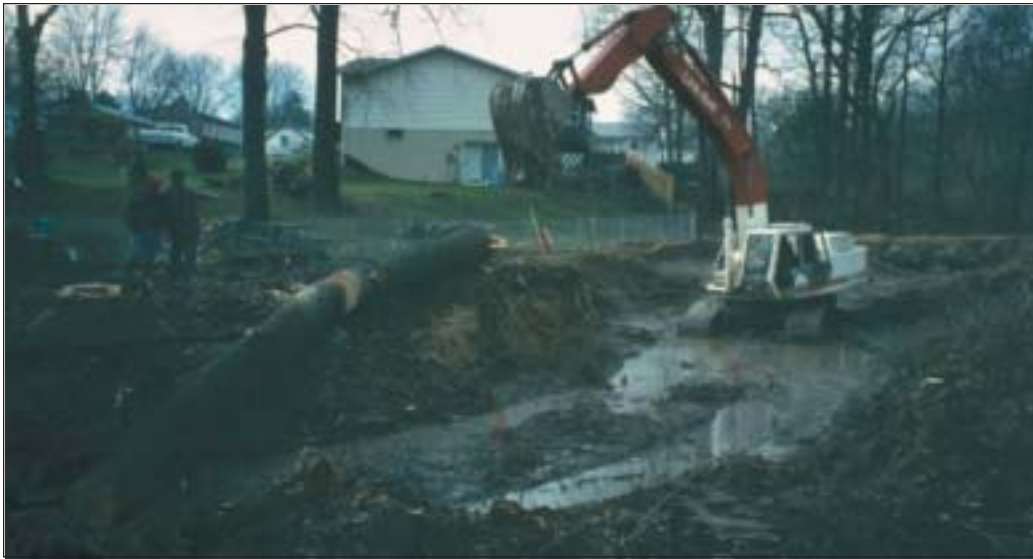
Bank stabilization activities in Tributary 9 during construction.
