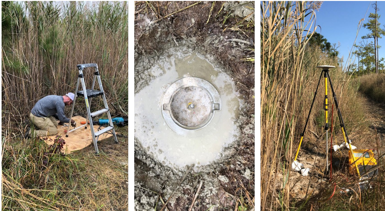
Figure 5. Installation and monitoring of the Peter's Neck survey mark (PTNK).
