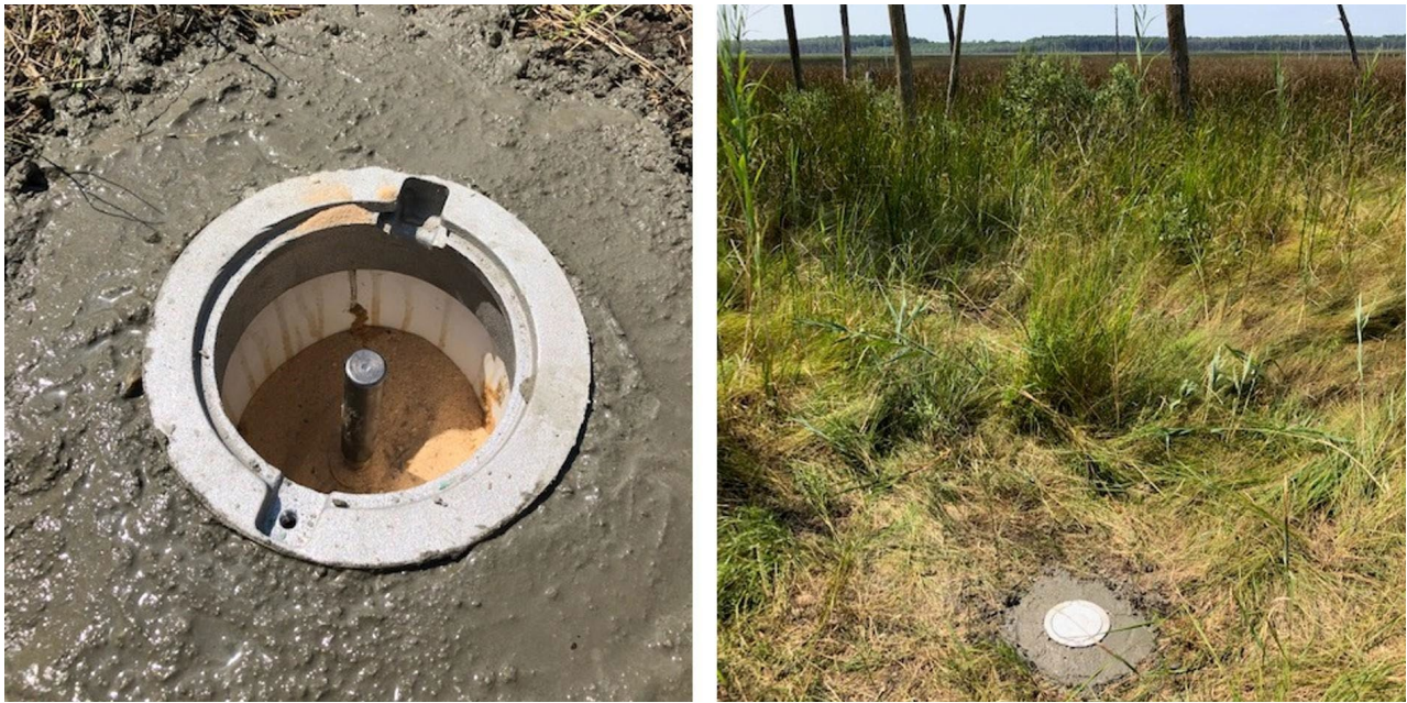
Figure 3. Installation of the Money Stump survey mark (MSTP).
